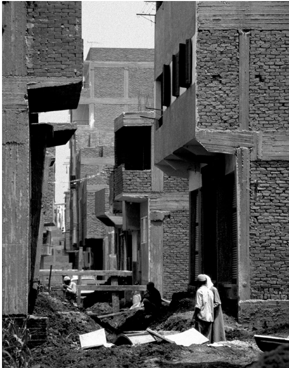
Informal housing under construction Dick Doughty/ Saudi Aramco World/PADIA
